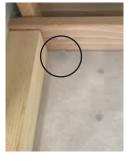
Here is an inner view showing the linking bar hole. It is positioned next to the headboard fixing holes push through from inside to create guides.
