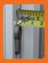
Step 2 - Measure how far lock protrudes, (see diagram) and select number of pads needed (1mm = 1 pad).
