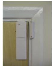
**NOTE:** The magnet must not be more than 1cm from the transmitter when the door is closed.
