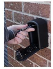
7.Finally use the socket driver to fully tighten all four fixings into position. You should find your Keyguard XL is firmly secured in position.
